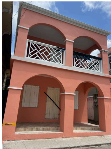
Savor St. Croix after renovations, made possible through the combination of EZC and EDB products.
