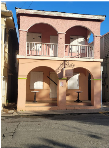
The site of Savor St. Croix before renovations.
